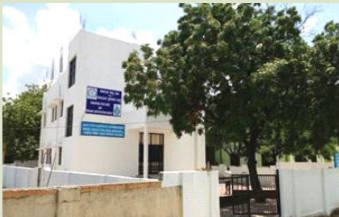
Seed Testing Laboratory and Training Complex at Raichur
